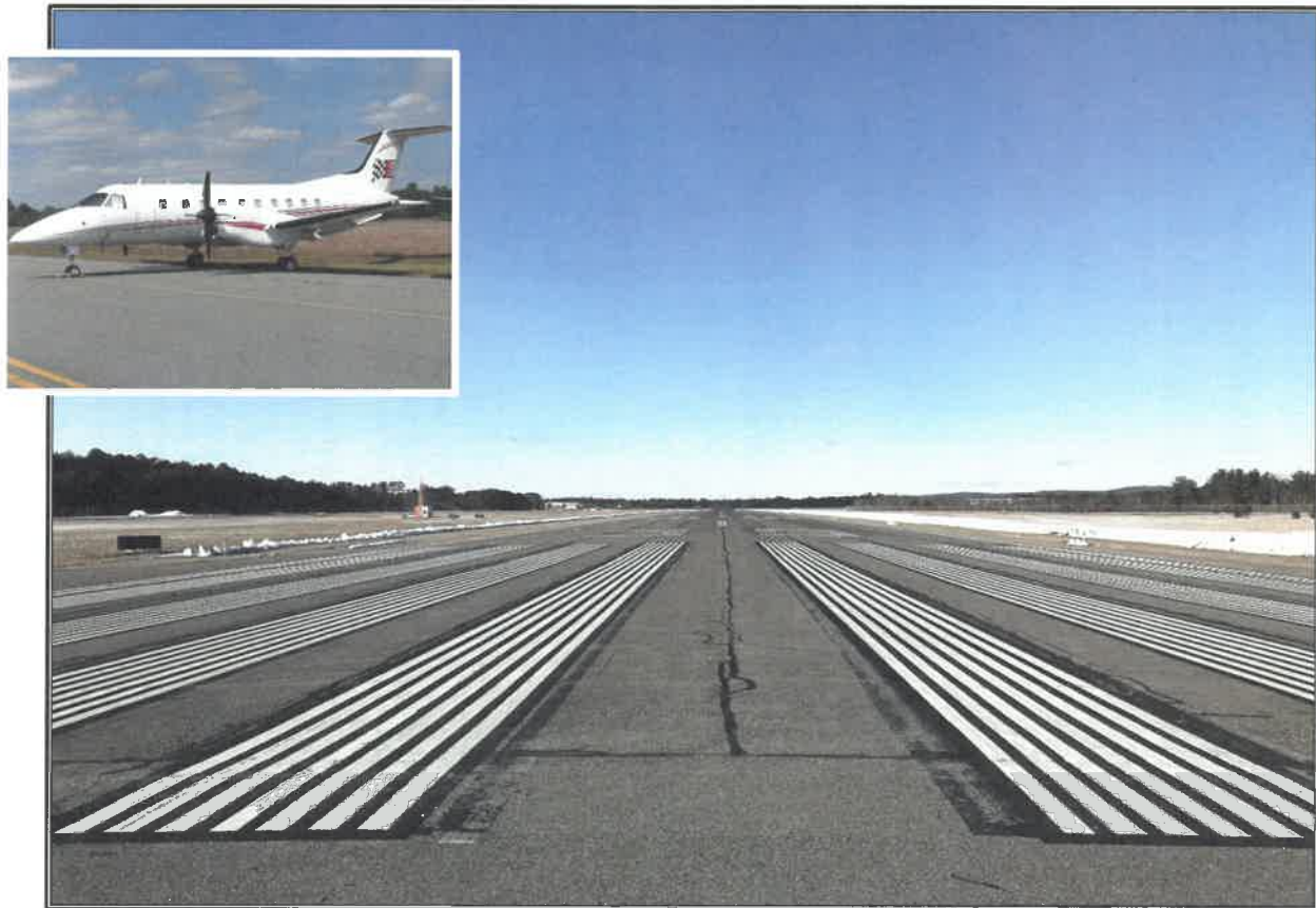
Figure 3: View of Concord Municipal Airport's Runway 17-35.
