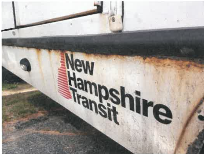
SCS: Corrosion on lower panel/wheel well
