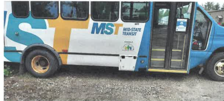
CAPBM: Corrosion on wheels and along exterior
